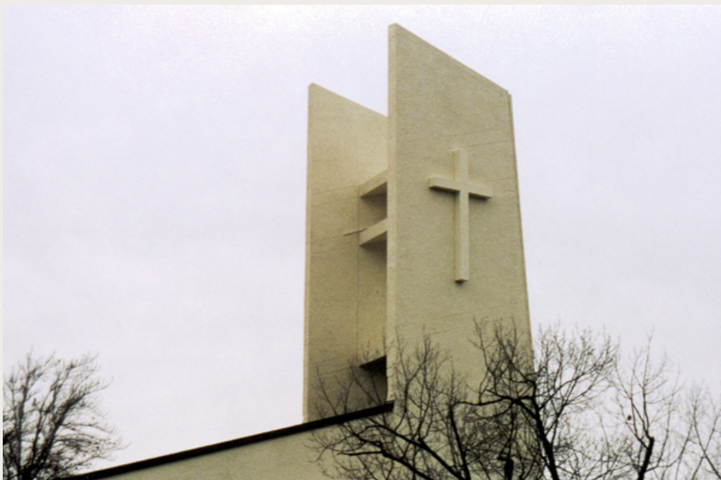
Figure 8: Cell tower disguised in cross by Larson Camouflage
